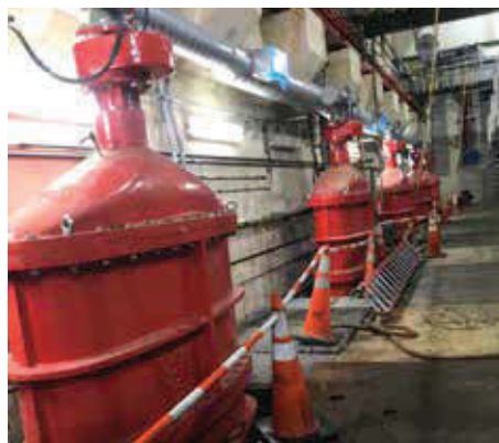
60" Resilient Seated Gate Valve. Made in the USA. Installed in Sayreville NJ
